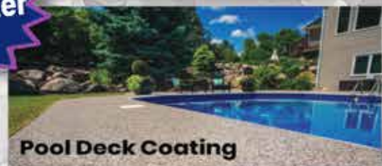
Patio Surface Coating
