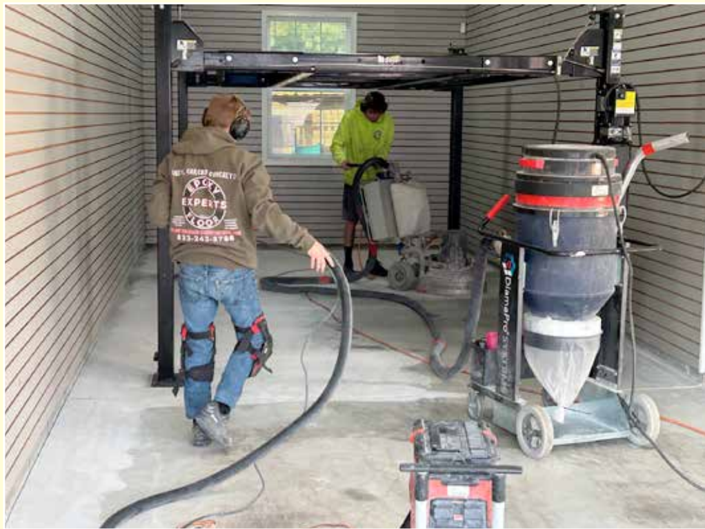
With D-day here the team of young men started off by Diamond cutting the entire 950sq foot concrete floor with industrial machines and smaller handheld versions to get in all the small and tight places.
